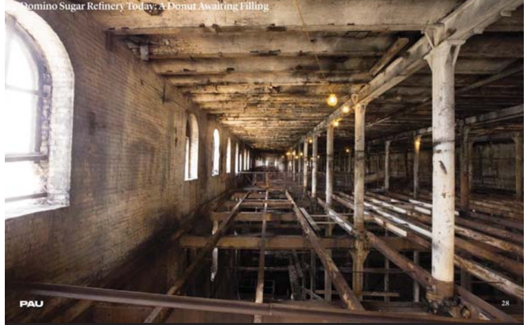
Domino Sugar Refinery Today: A Donut Awaiting Filling
